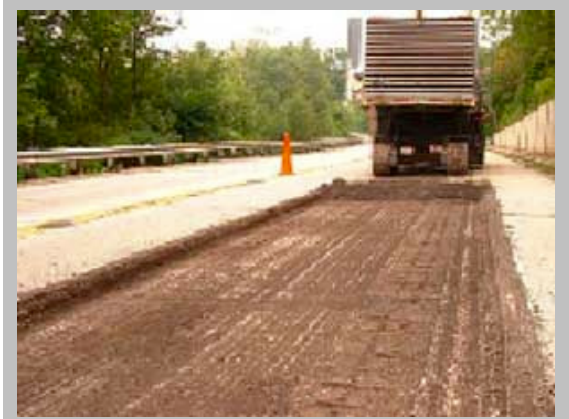
One FFY 2008 project for the Flexible Pavements will study pavement repair prior overlay, such as base patching.
