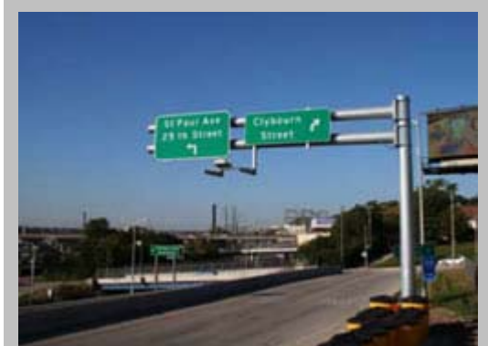
Researchers are assessing the fatigue-induced fracture risk of sign support structures like this one off I-94 in Milwaukee.
